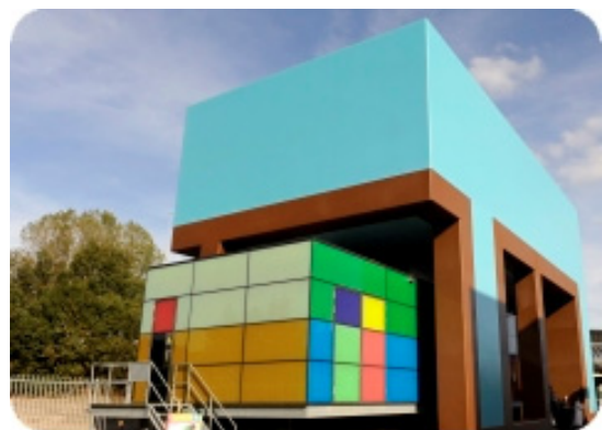
Amsterdam RAI Substation
